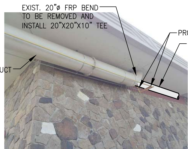
NEW 10" FRP CONNECTION TO EXIST. 20" FRP DUCT
