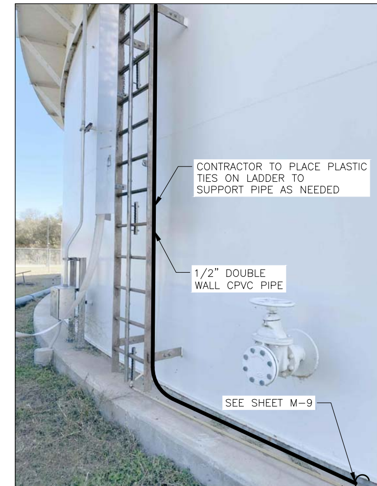
6 APPROXIMATE PIPE LOCATION
