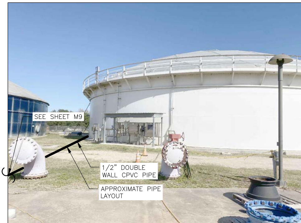
5 APPROXIMATE PIPE LOCATION
