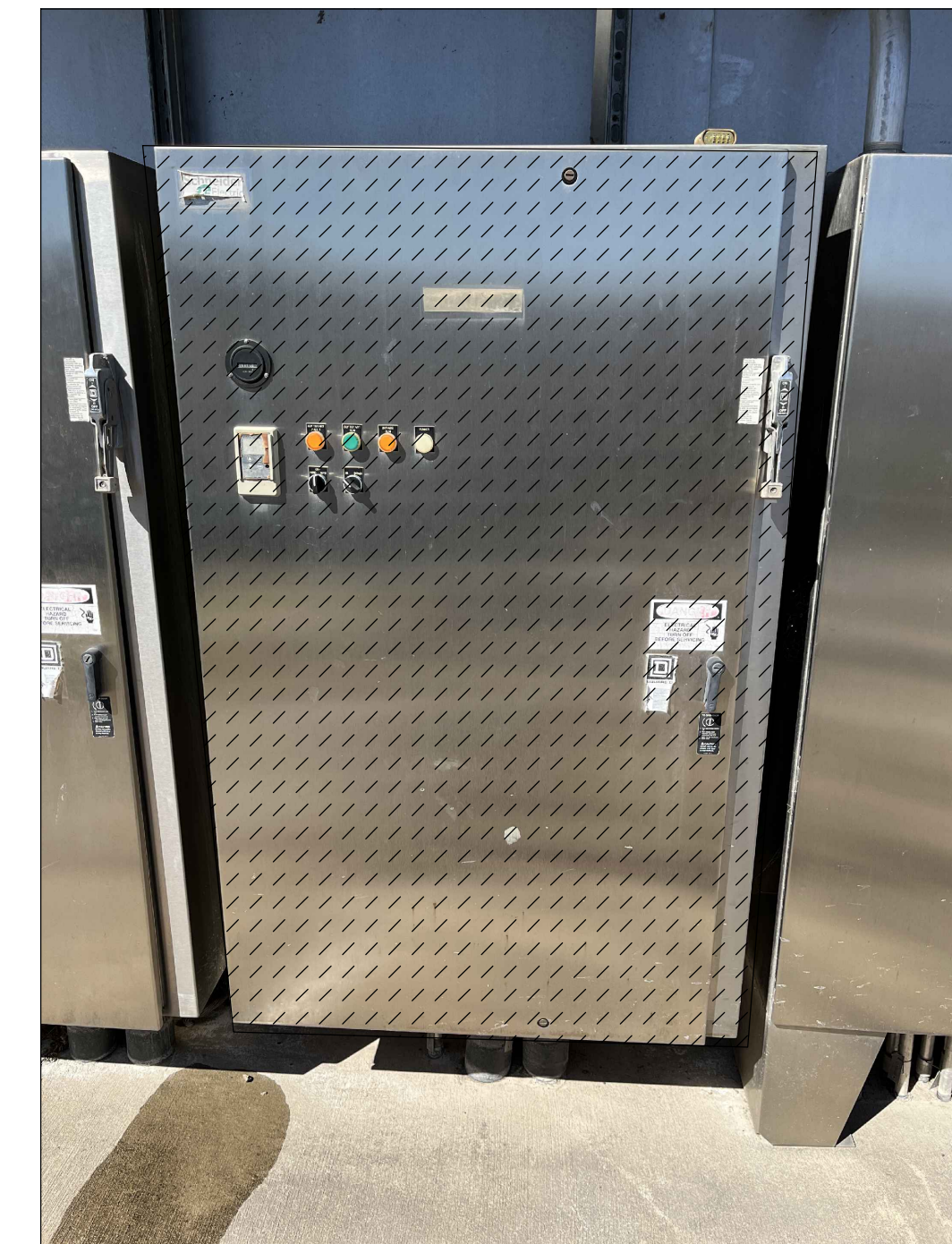
IWP-03 STARTER DEMOLITION PHOTO 3 NTS
