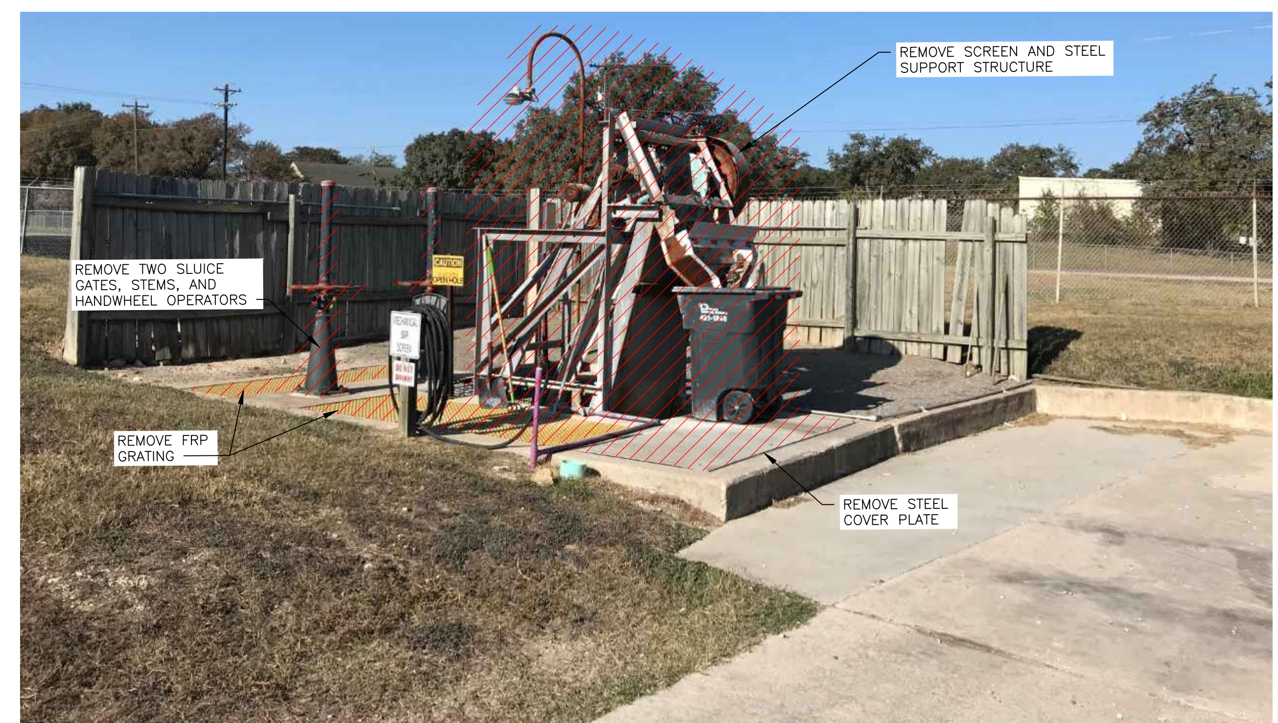
BAR SCREEN DEMOLITION DETAIL PHOTO NTS
