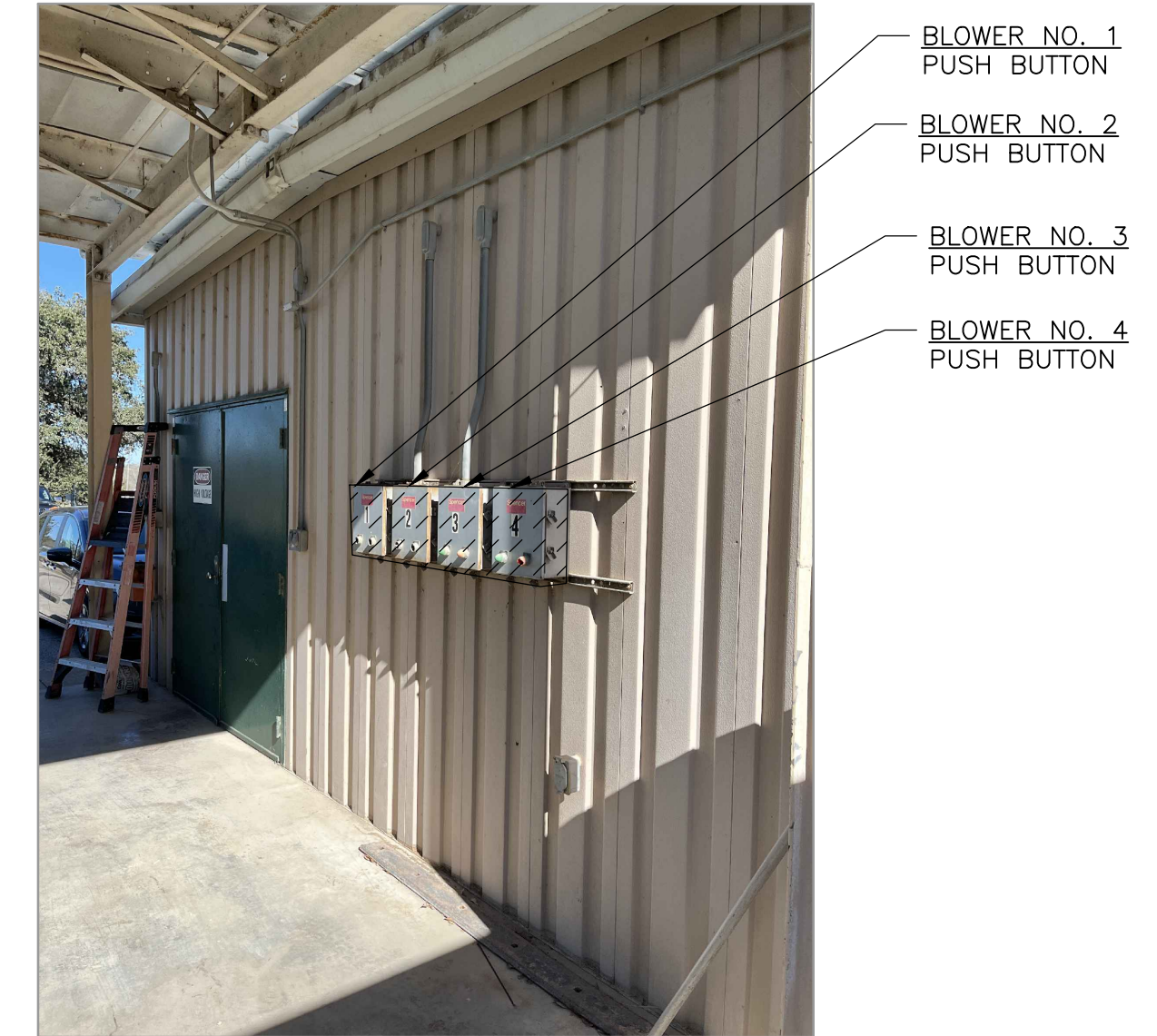
BLOWERS PUSHBUTTON DEMOLITION PHOTO 2 NTS
