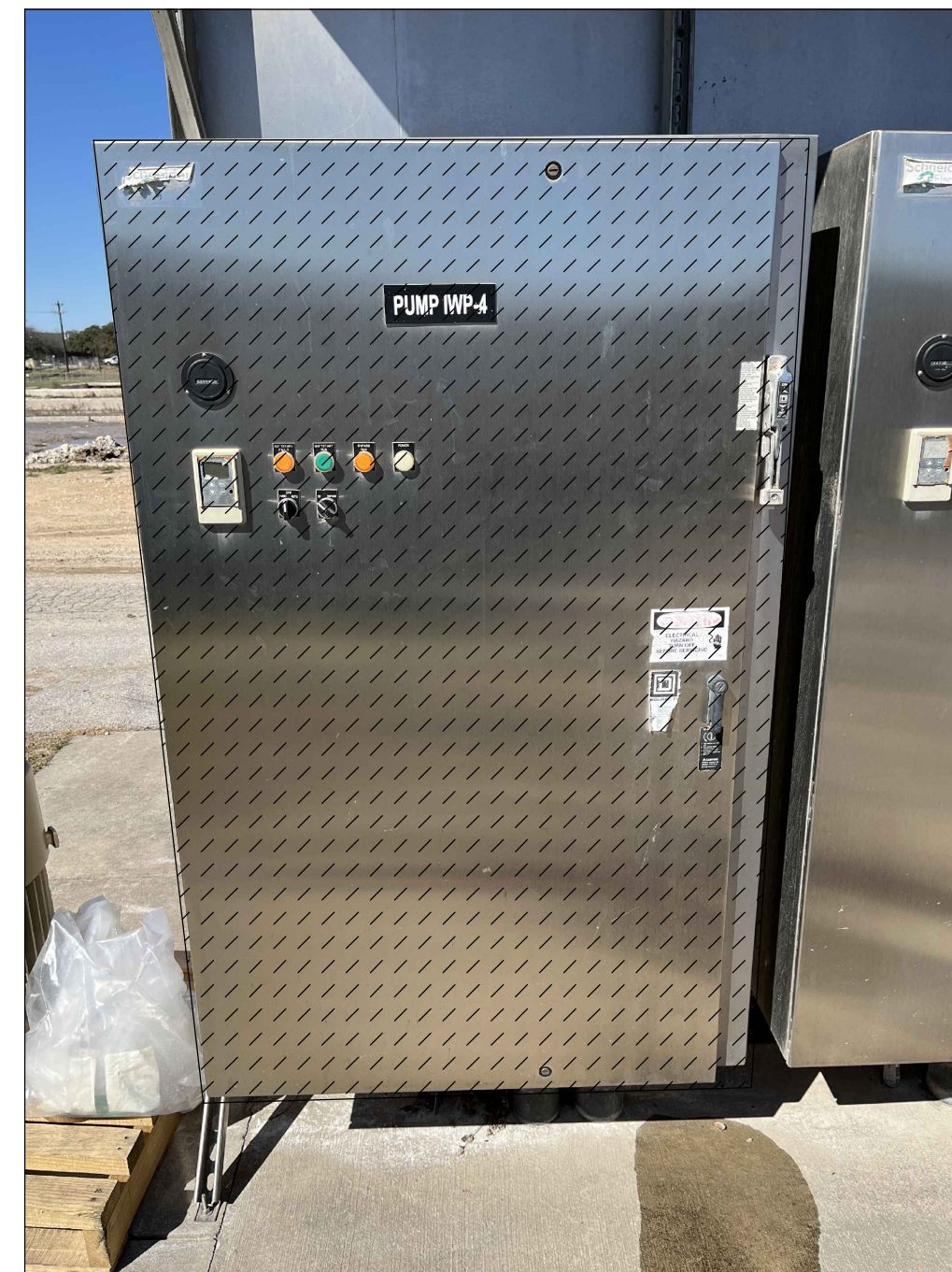
IWP-04 STARTER DEMOLITION PHOTO 4 NTS
