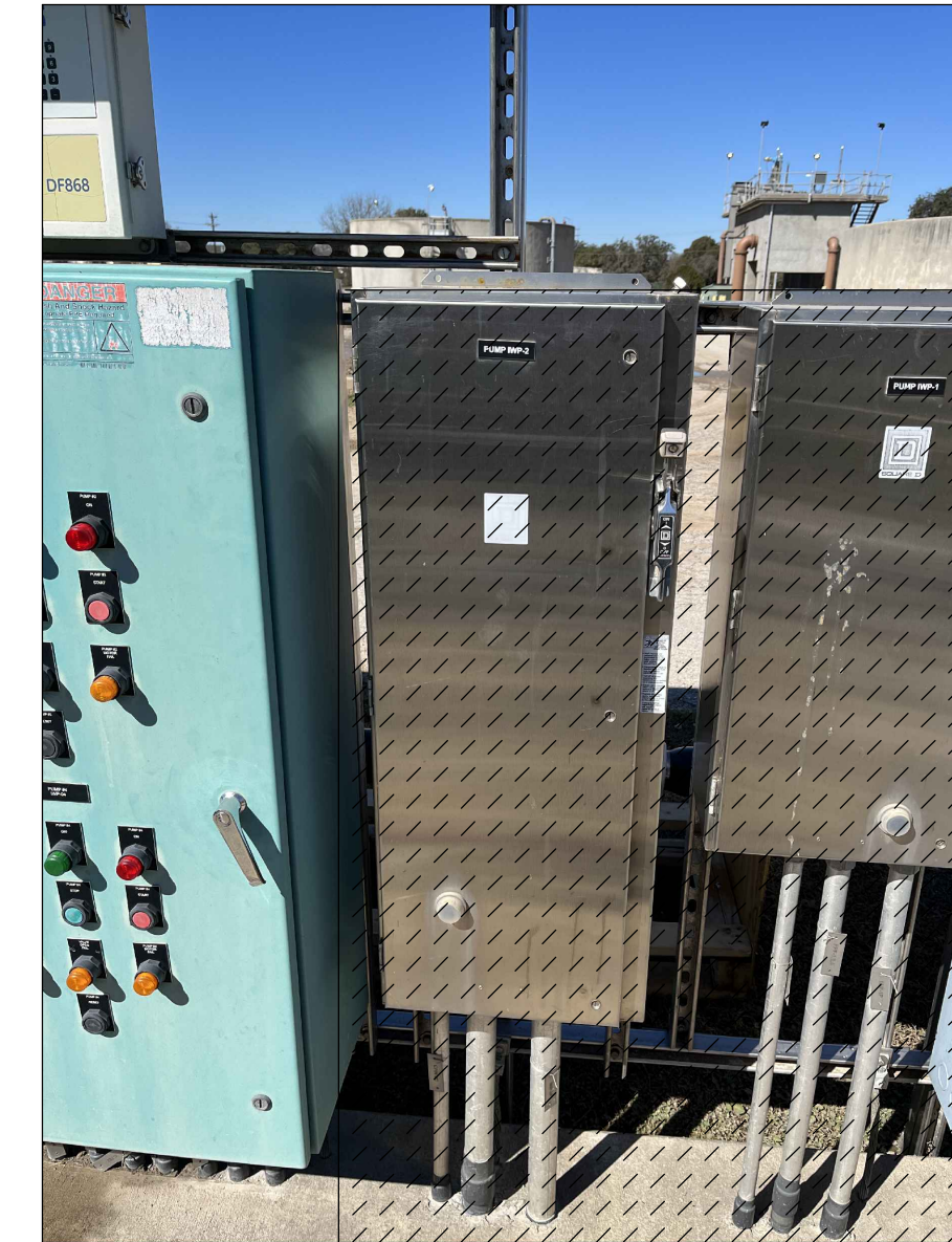
IWP-01, 02 STARTERS DEMOLITION PHOTO 2 NTS
