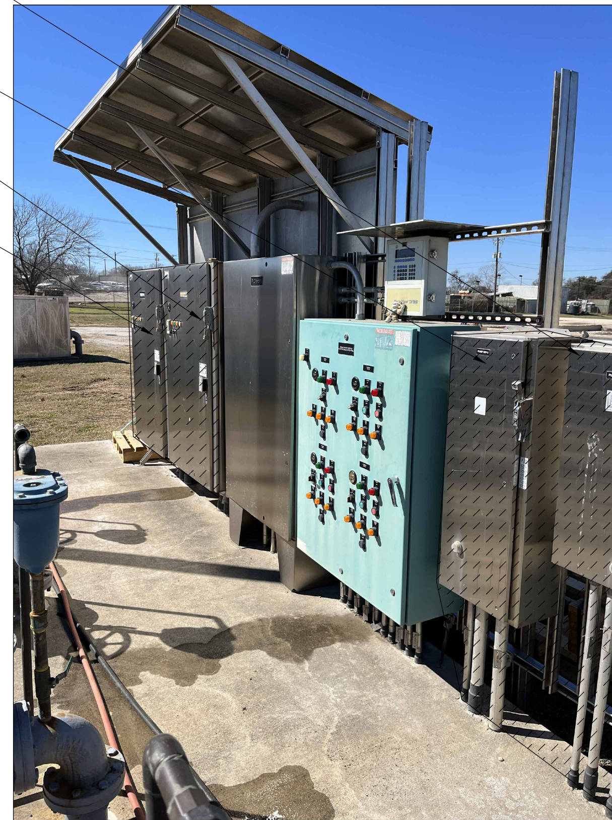
DEMOLITION PHOTO 1 NTS
