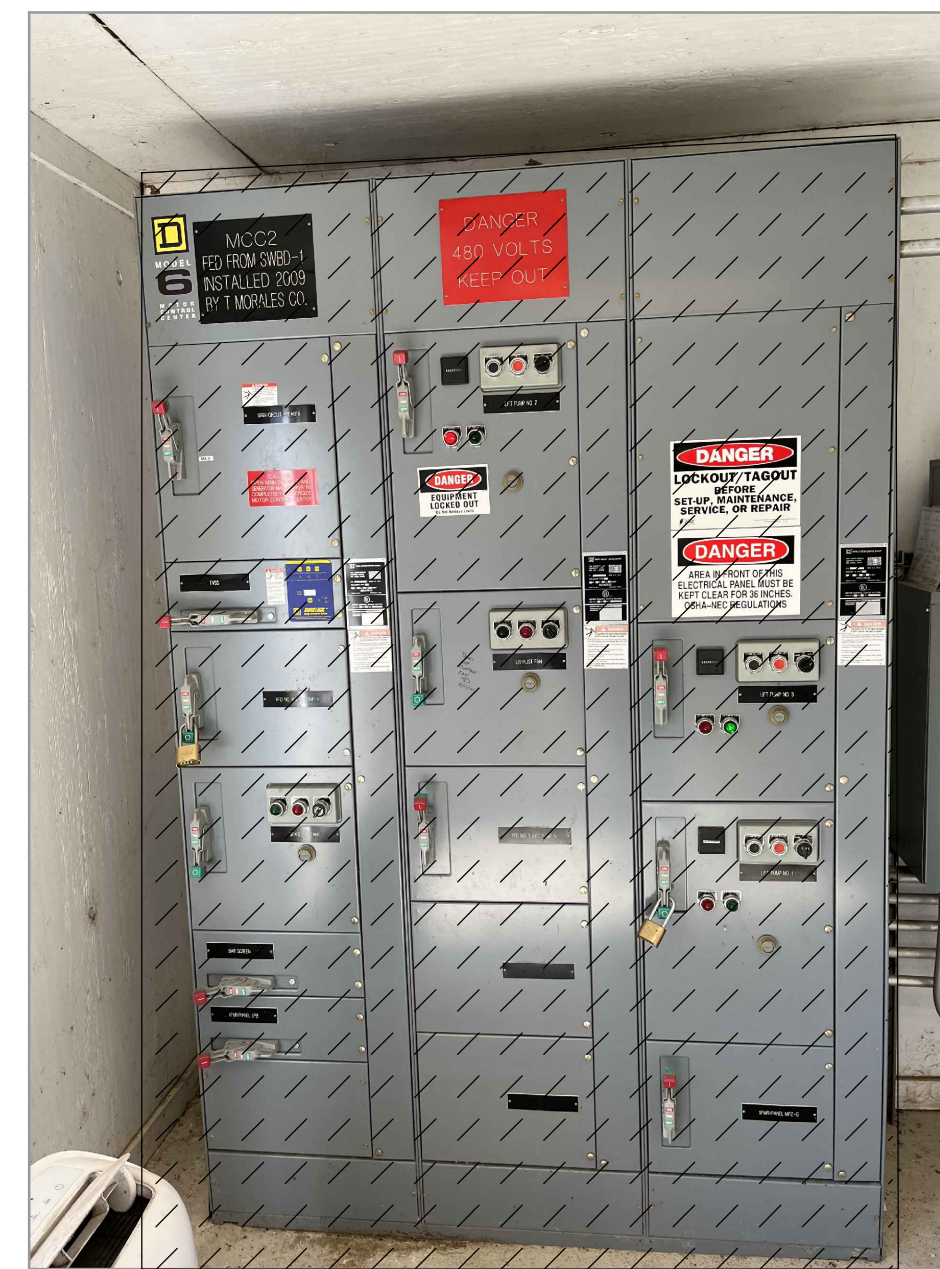
EXISTING MCC-2 DEMOLITION PHOTO NTS
