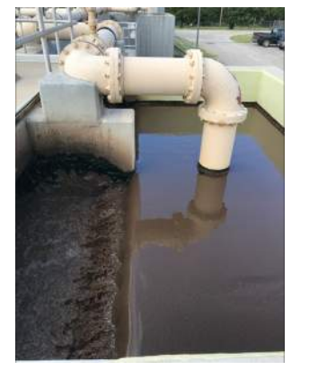
PHOTOGRAPH OF AERATION BASIN INFLUENT WEIRS TYPICAL FOR AERATION BASINS 1/2 AND 3/4
