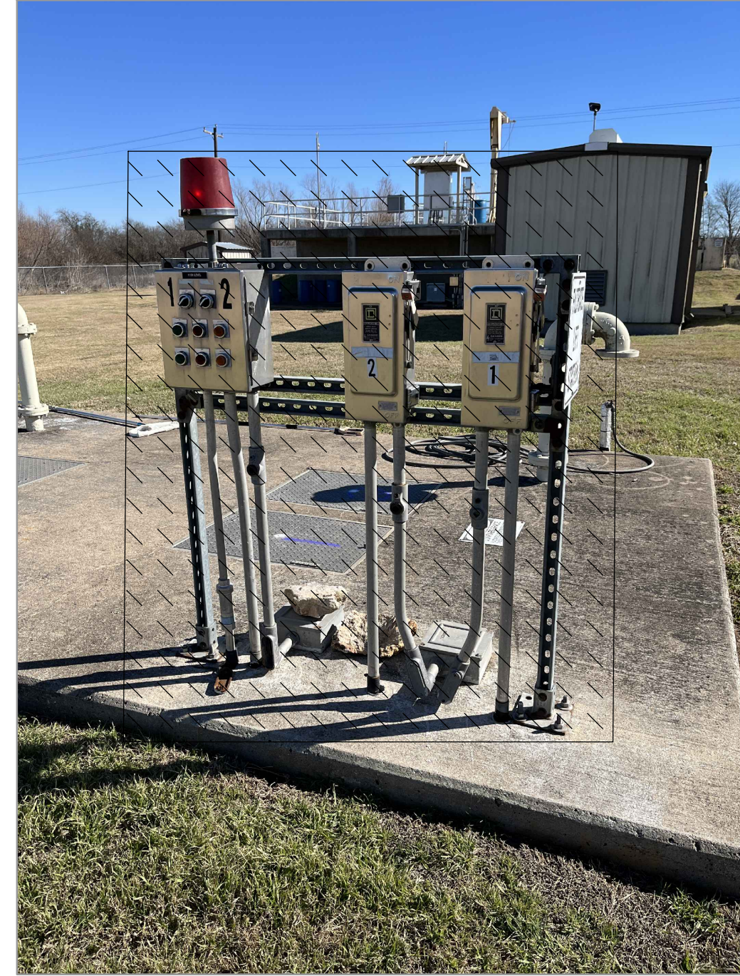
DEMOLITION PHOTO 1 NTS
