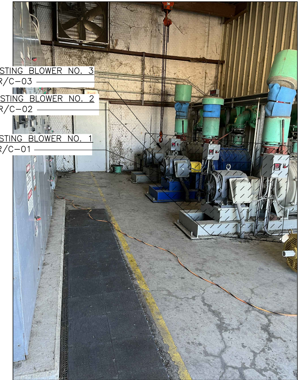
EQUIPMENT DEMOLITION PHOTO 1 NTS
