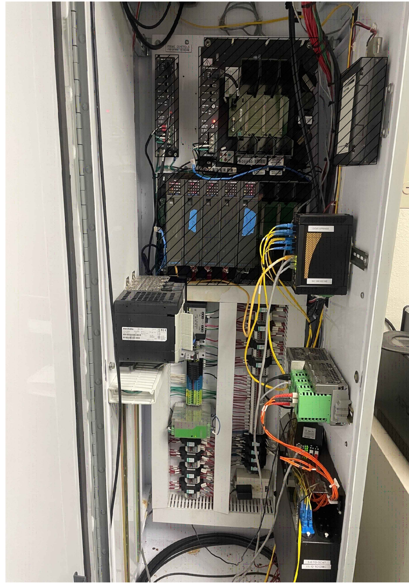
RTU-DSWTP PANEL MODIFICATIONS
