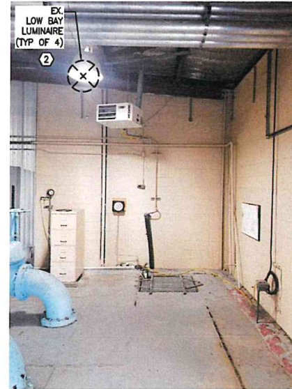
3 LOW BAY LUMINAIRE ② E2.2 SCALE: NTS
